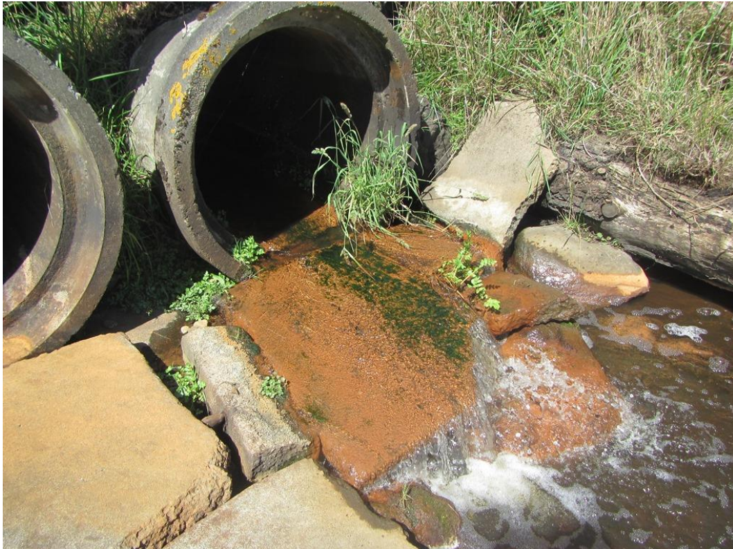
Plate 11: Culvert pipe being a partial impediment to fish passage in the channel downstream of the Pukepuke Conservation Area. 15 March 2017.
